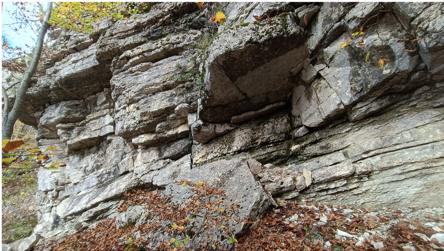
Fig. 5. Field picture of the Bugarone Inferiore Formation in Pian del Sasso. At the bottom right is the stratigraphical contact with the greenish-grey nodular limestones belonging to the Rosso Ammonitico Formation (Upper Toarcian). The lower Bajocian block of nodular limestone from which the described ammonites come has detached from the wall at the top left of the photo.
